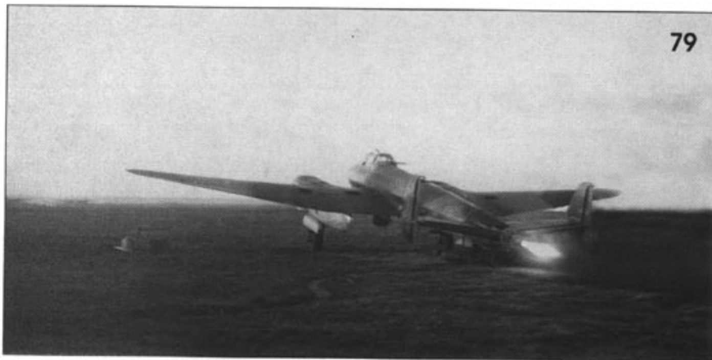
79. Наземные огневые испытания самолета Пе-2 с ускорителем РУ-1 на аэродроме в Казани. Ground firing of a Pe-2 equipped with the RU-1 rocket booster being conducted at an airfield near Kazan'.
